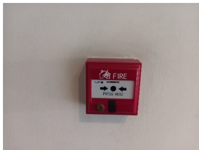
Fire Alarm Manual Station
